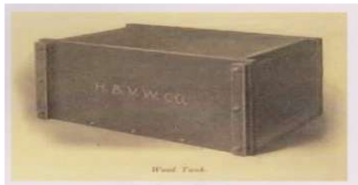
Fig. Wood Tank
