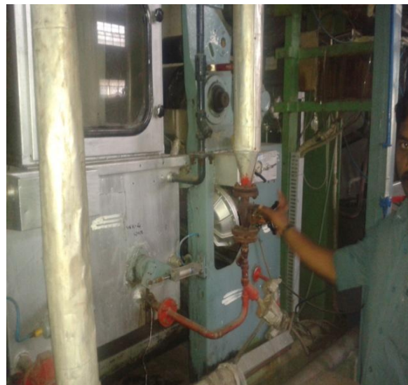
Open the steam, air and water valve
